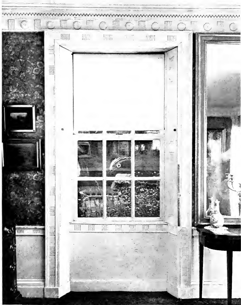
PLATE CVIII.—Detail of Embrasured Window, East Parlor, Pierce-Johonnot-Nichols House.
